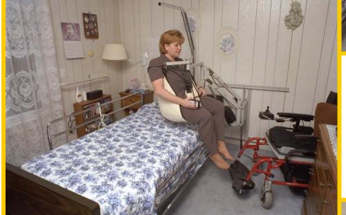
◆ The lift is powered by a transformer at each wall mount station
